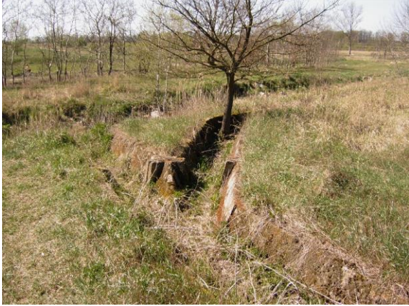
Trickle field around Berlin with ditches (wastewater disposal & reuse on agricultural fields)
